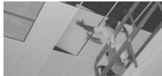
Duro-Therm panels used in a ceiling.
